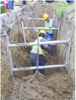
3. Shielding protects workers by using trench boxes or other types of supports to prevent soil cave-ins.
