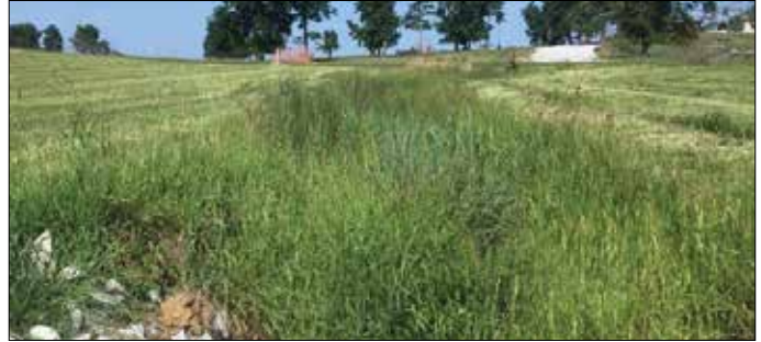
Figure 5. Vegetative strips in combination with weirs slow water and reduce erosion.
