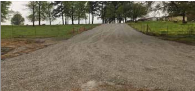
Figure 6. A major travel corridor for animals and equipment was reinforced.
