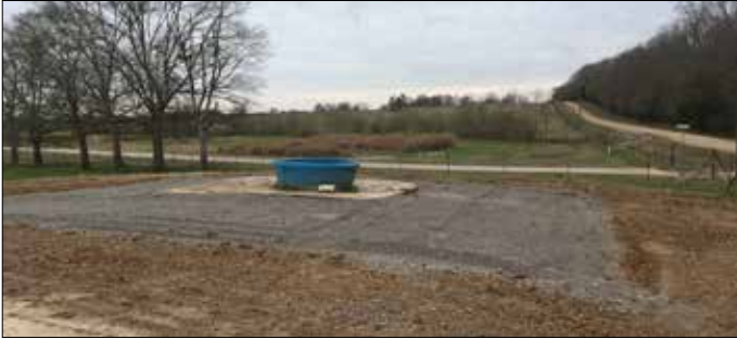
Figure 4. Heavy use pads under water troughs allow water to percolate through the gravel and geotextile cloth surface and keep livestock out of mud.
