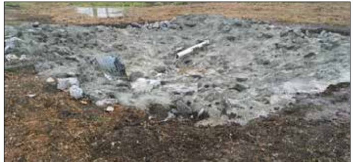
Figure 7. An area under a drainage pile was reinforced to stop erosion.
