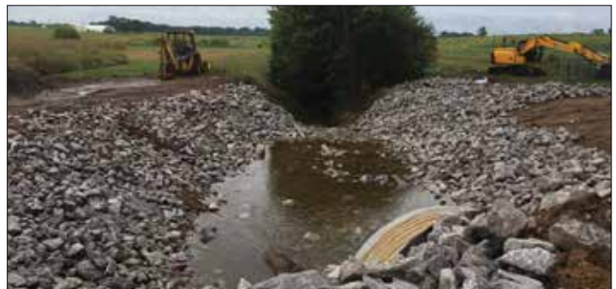
Figure 9. Bank conditions after installation of streamside stabilization practices.
